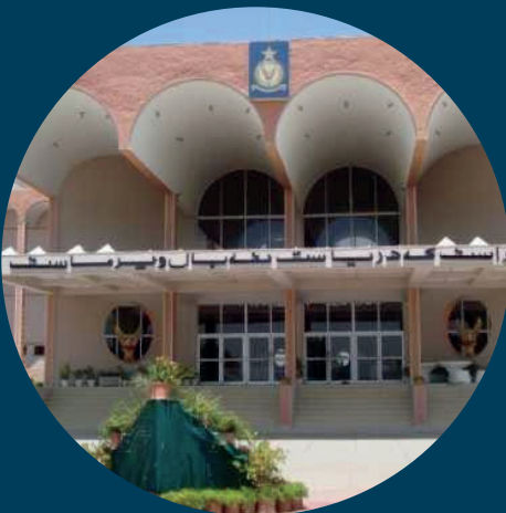
PAF Risalpur Waterproofing
