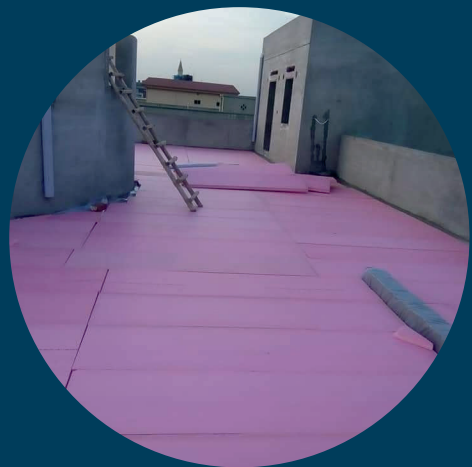
Residential Project 2 Heat Insulation
